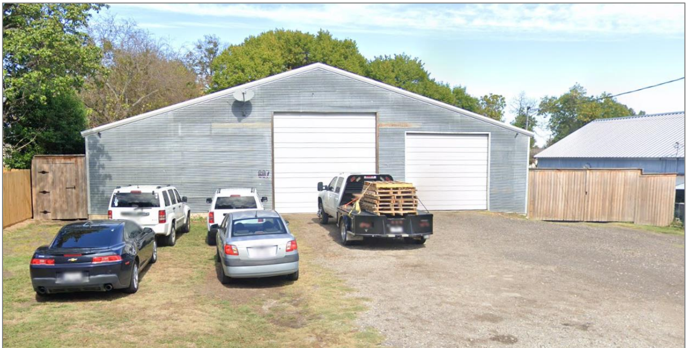
FIGURE 1: UNPERMITTED WOOD FENCE ON THE SUBJECT PROPERTY.
